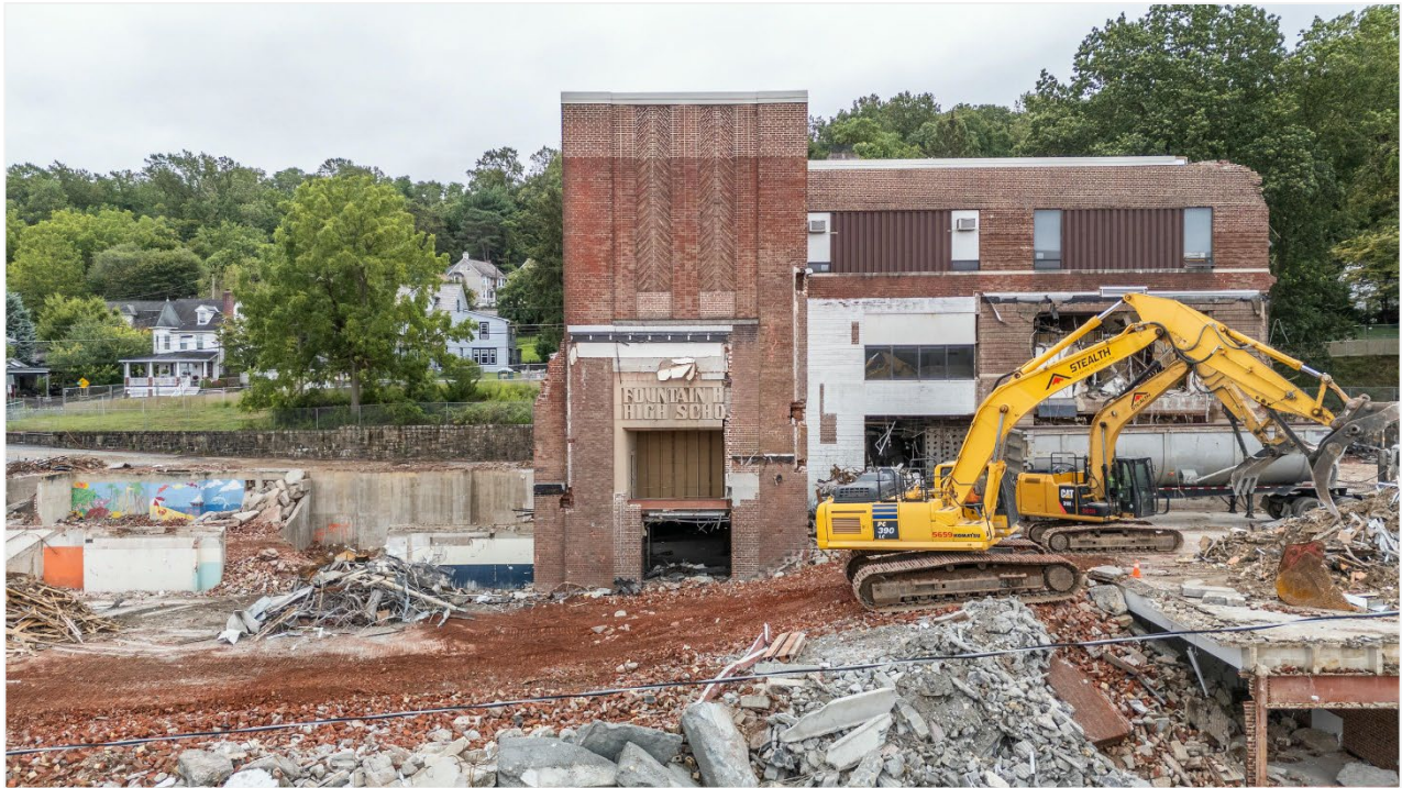
Continued Demolition of the Gymnasium
