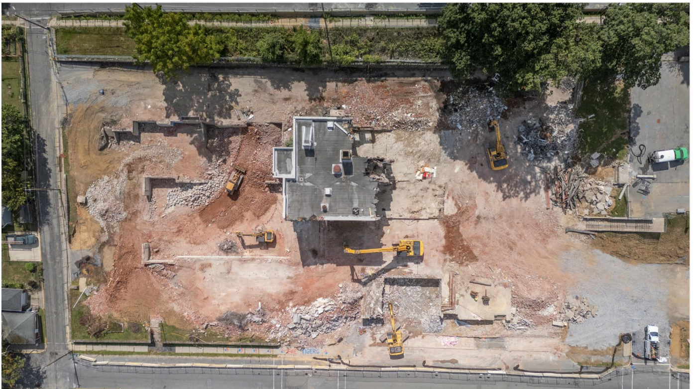
Drone View of Building Demolition August 28, 2025
