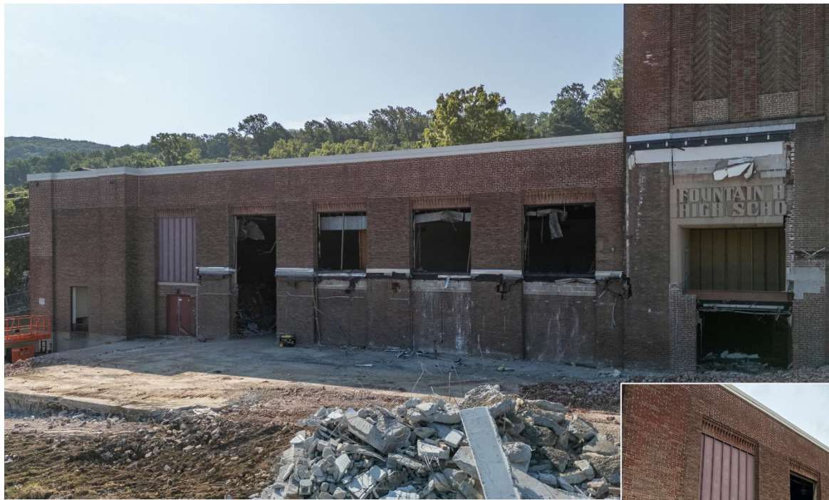
Demolished Administrative Office Area
