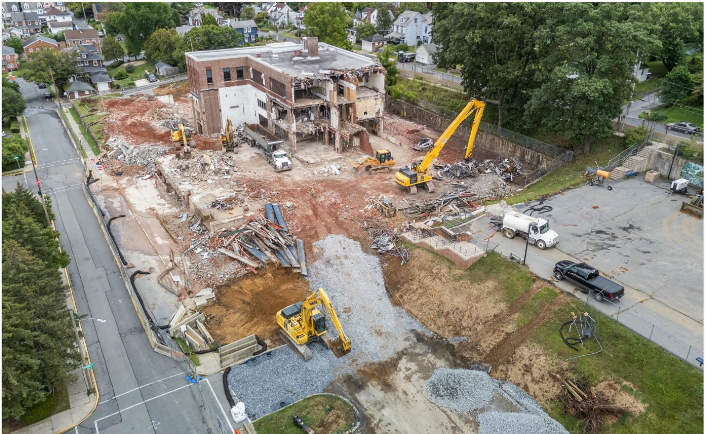
Drone View of Demolition of the Northwest Corner of the Building
