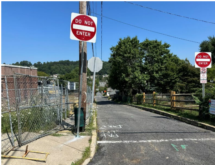
Traffic and Pedestrian Signage Installed on Garden Street
