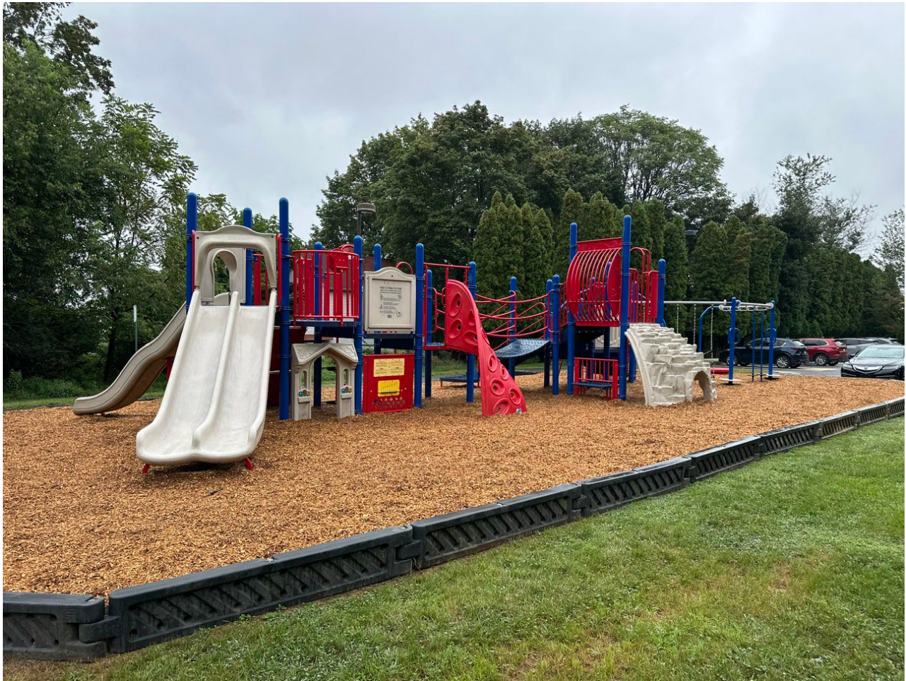
Playground Relocation and Mulch Installation Complete at Donegan Elementary School
