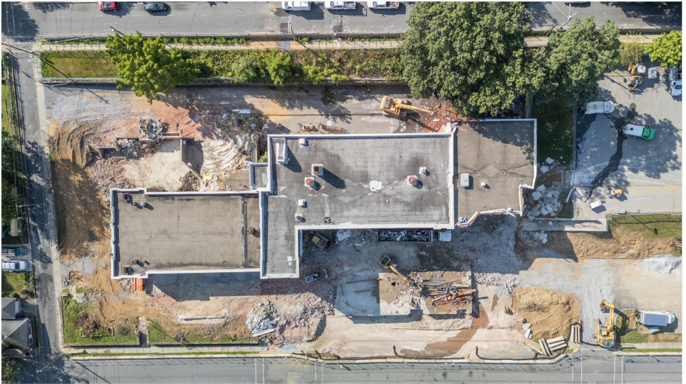
Drone View of Building Demolition August 11, 2025
